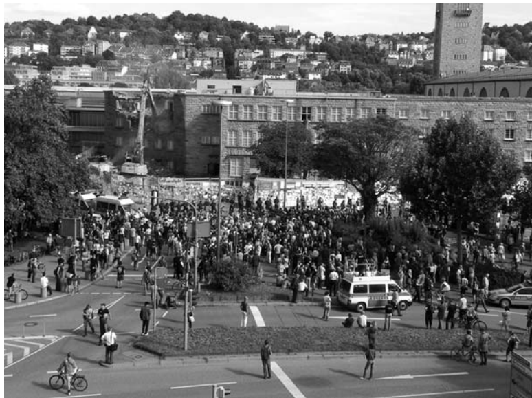
Figure 4. 25 August 2010. Demolition works begin in earnest at Stuttgart's Central Station. (Photo: Dirk Haun)
